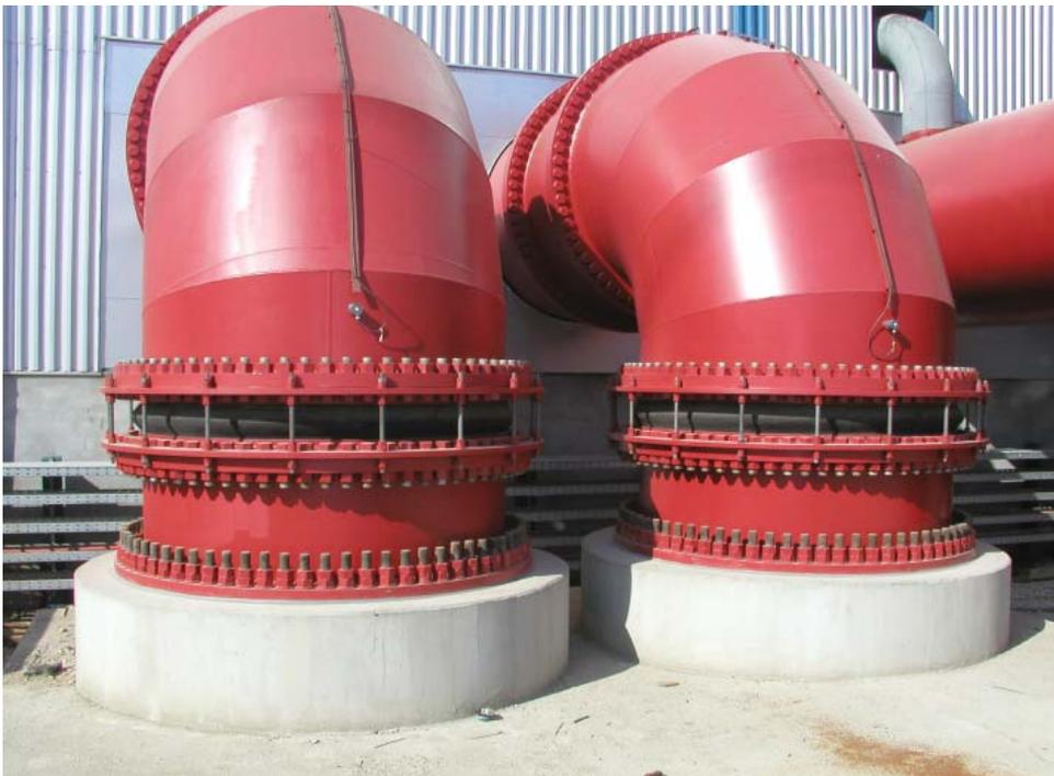
restraint compensator - design M DN 2600
